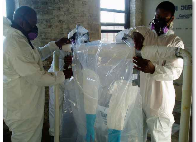
People at work removing asbestos PHOTO – greenforall.org / CC, Flickr
